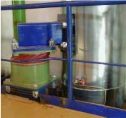
*Fig. 1 VD-Damper Installed on Pipeline of NPP (Turbine Hall)*
